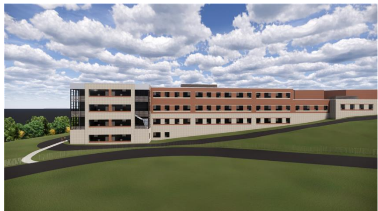
Top: Aerial view of the future Staunton High School.
